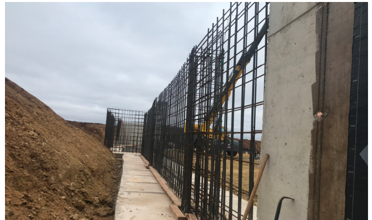
Rebar Tying at North Gym Retaining Wall
