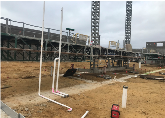
Area B and C Inwall Plumbing Rough-ins
