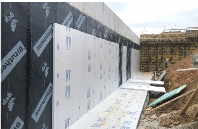
Waterproofing – West Gym Retaining Wall
