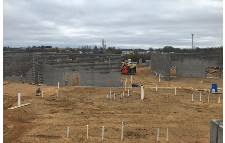
Area B & C Underground Plumbing
